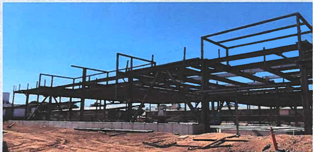
View from Valley/3 rd Staff Parking Lot
