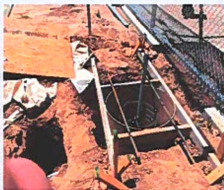
Light Pole Foundation
