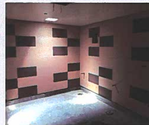
Student Toilet Room
